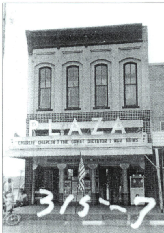
Figure 14: Paschall Building Source: 1946 city tax records, Denton County
