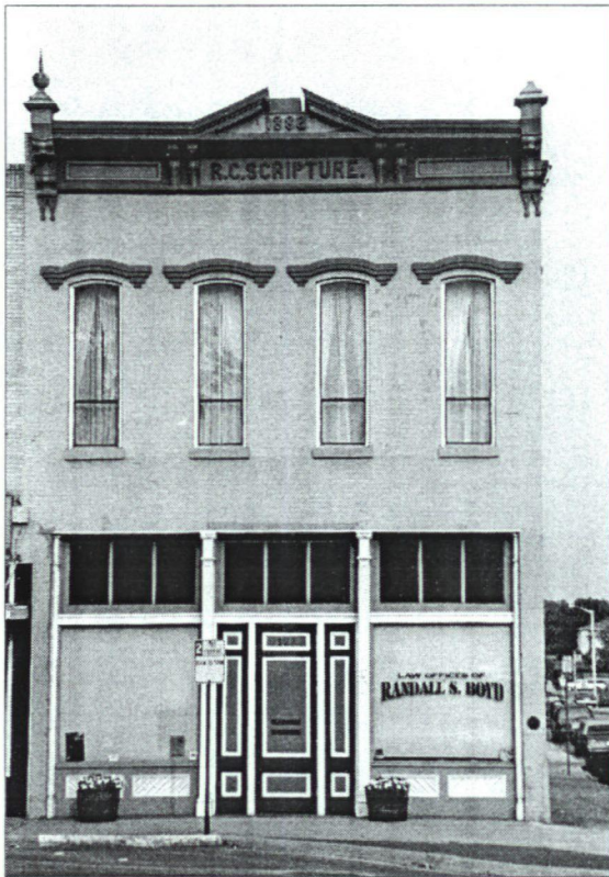
Figure 12: Scripture Building (123 North Elm) Source: Knight and Associates
